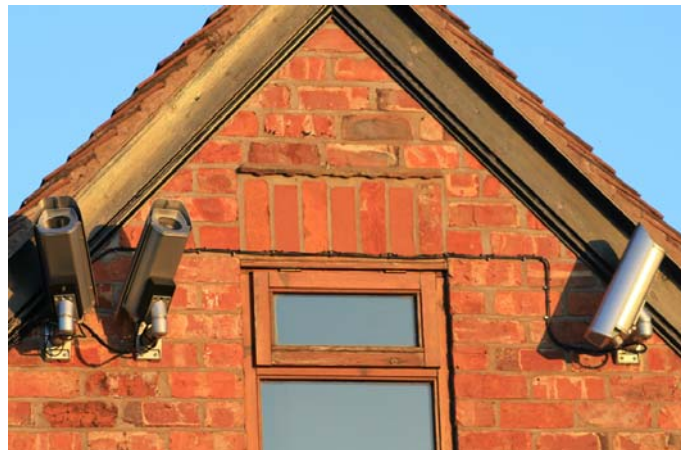
Figure 1. The three cameras of the Ravensmoor node permanently affixed to the gable end of a brick building. The unit on the left faces southeast, the middle one northeast while that on the right faces north. Note the black spacer block on the first two units between the camera housing and the mounting bracket. This modification was required in order to allow the appropriate elevation to be achieved without the rear of the housings fouling on the horizontal support bracket.
